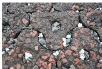
Holes in revetment stones to attract marine organisms. Source : EcoShape
