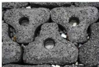
Holes in revetment stones to attract marine organisms. Source : EcoShape
