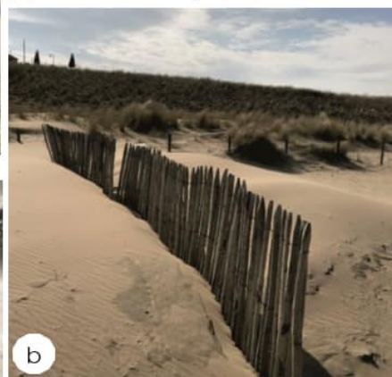
(a) Brushwood fence (b) Vertical planks fence (c) Perforated recycled plastic fence
