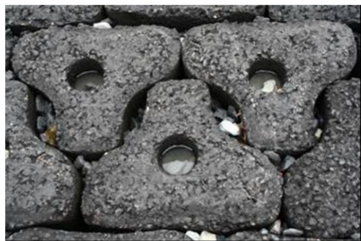
Holes in revetment stones to attract marine organisms.
